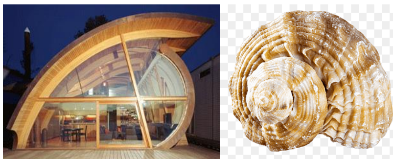
Figure (7) Shows Fennell Residence Project
