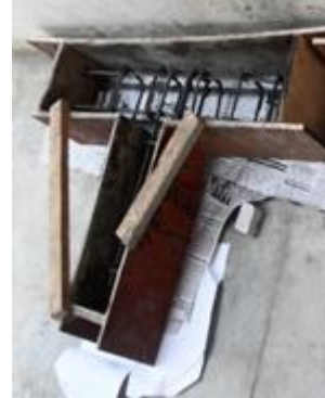
Figure.4 Beam Column Joint- Reinforcement
